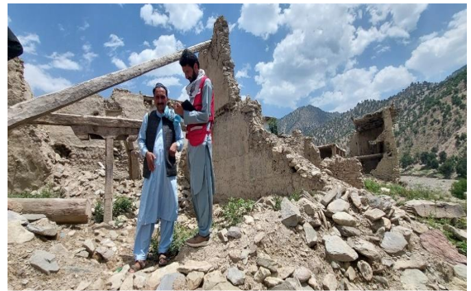
ARCS engineers carrying out shelter damage assessment in Spira district of Khost province. (Photo: ARCS)
